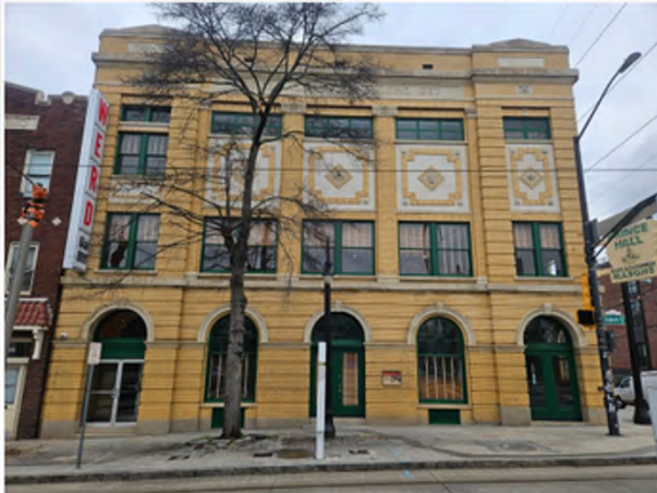
Former offices of SCLC/MLK Jr. Most Worshipful Prince Hall Grand Lodge of (Atlanta) Georgia
